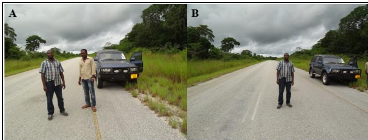
Figure 2: Photos showing access to the project area. A and B well maintained bitumen road of southern corridor connecting Mtwara port to project area.
